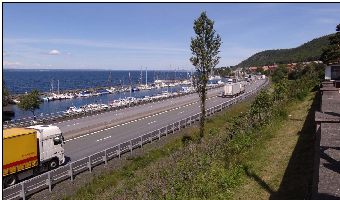
Figure 1 – The motorway E4 between Lake Vättern and a residential area in Huskvarna, Sweden.
