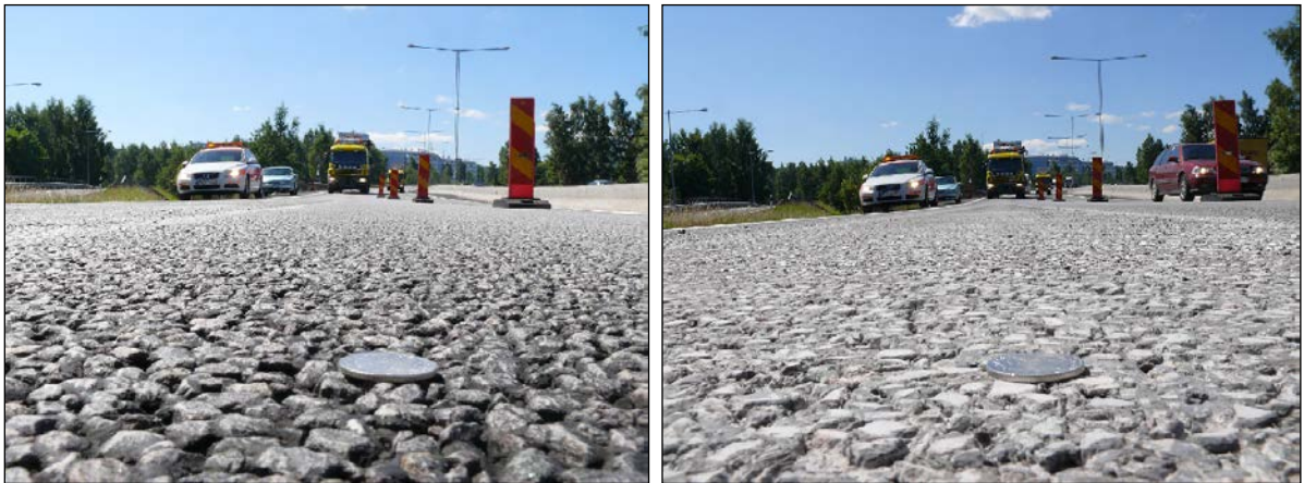
Figure 11 – Non-ground surface (left photo) and ground surface (right photo). The coin diameter is 25 mm.
