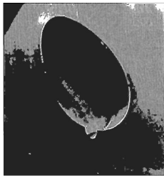
Figure 2. A speaker unit, mounted in the exhaust stack (view from inside the exhaust stack). Note the spout at the bottom to drain any residual liquid after cleaning.
