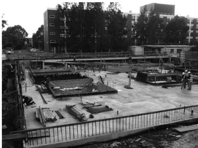
Figure 4: Site layout during construction showing laboratories (with isolated masonry walls) with isolated slabs yet to be poured.
