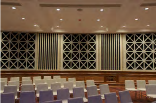
Figure 2. Installed acoustic diffuser panels and displacement air grilles, with architectural facings
