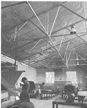
Richmond Technical School's Panel Shop with its RIPPLE SOUND ceiling
