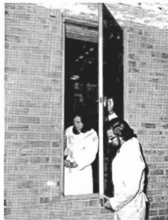
Fig.6. Framed door panel sheathed both sides with hardboard bonded to sheet lead.
