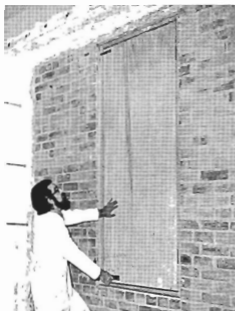
Fig.5. Door and frame installed in brick wall.
