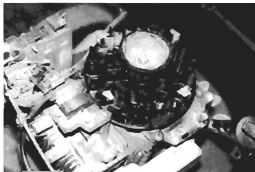
Figure 2. Top of motor with fan cover removed showing reflective strips on the motor fan.
