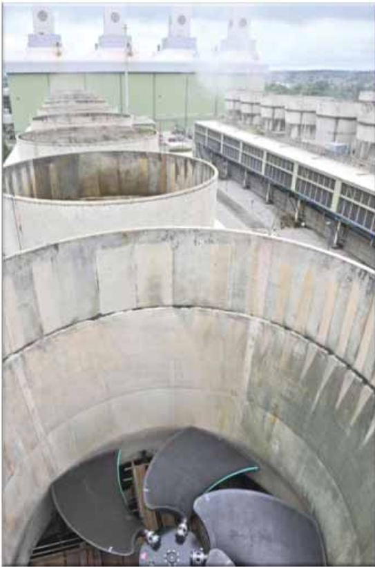
Figure 3. SX fan instead of the attenuation baffles.
