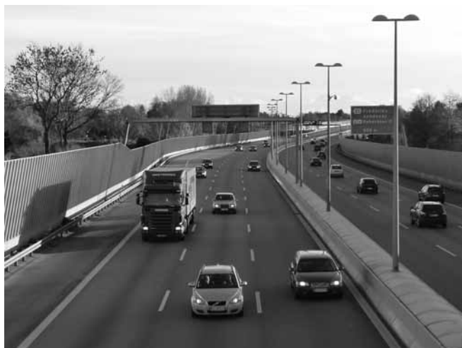
Figure 2. The M3 highway once completed, with porous asphalt and tilted 3m and 4m noise barriers.
