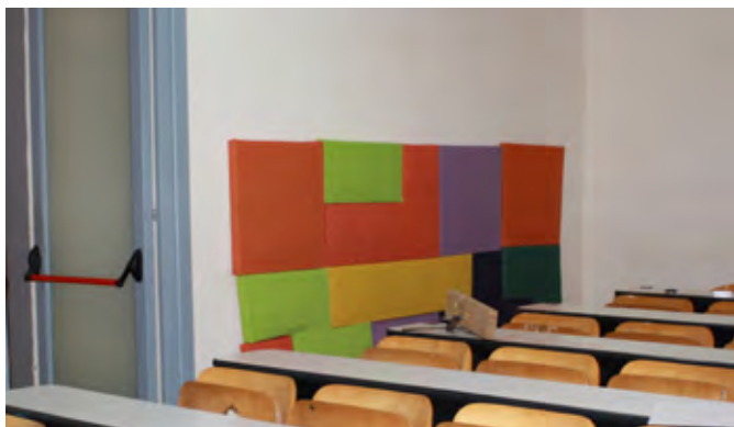
Figure 12. Sound absorbent panels inserted in a classroom
