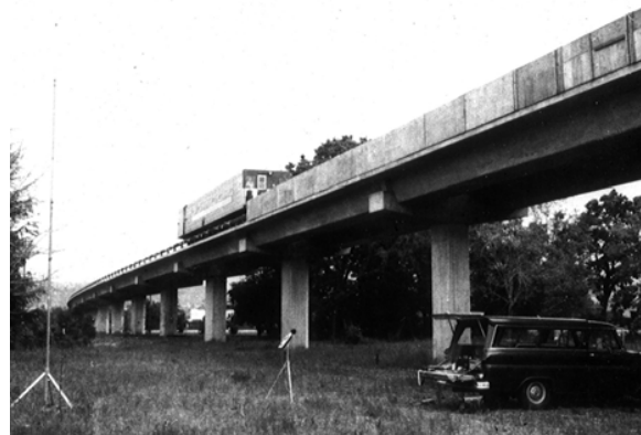
Figure 2 Photo of BART Test Track concrete viaduct and trial sound barrier wall
