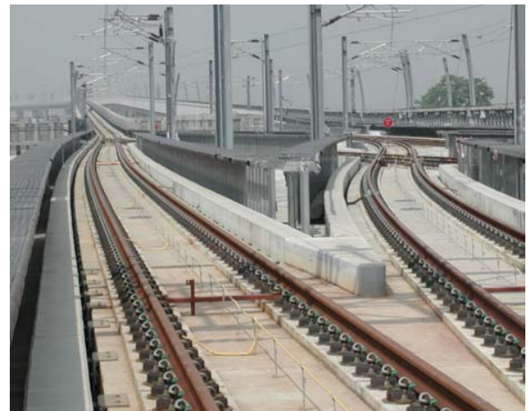
Figure 10 Photo of KCRC viaduct completed
