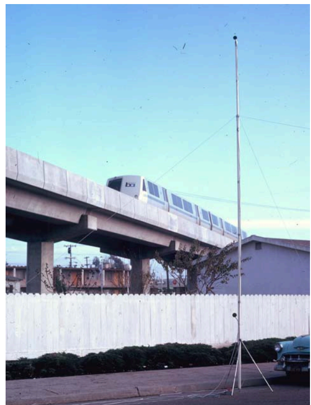
Figure 4 BART concrete viaduct with sound barrier wall
