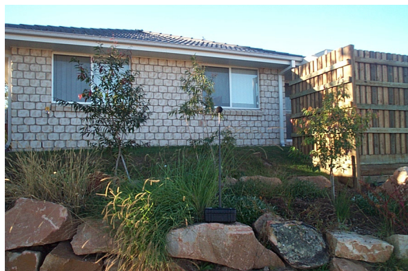
Figure 3. Noise Logger In-front of the Screen
