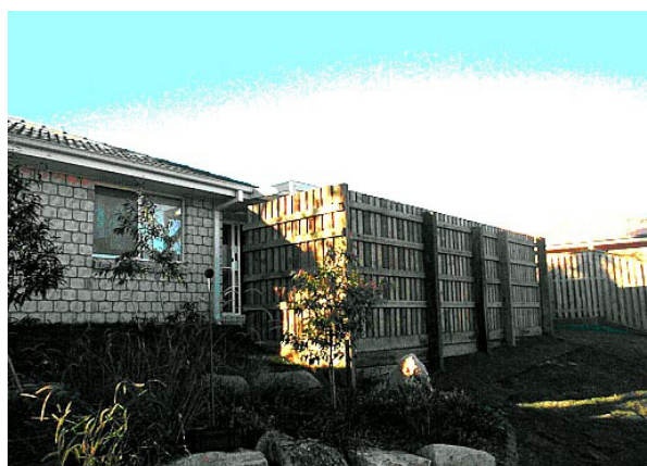
Figure 7. Acoustic Screen (As Constructed)
