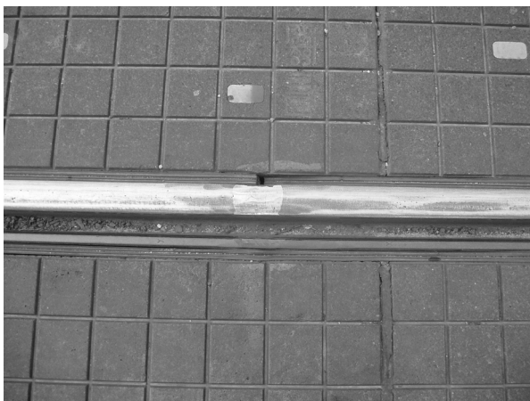
Figure 14b. Repaired rail weld - Location A
