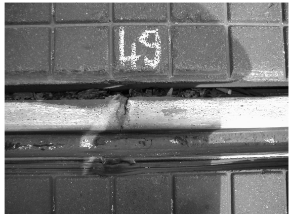
Figure 13a. Picture of weld - Location B
