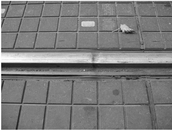
Figure 14a. Unrepaired rail weld – Location A
