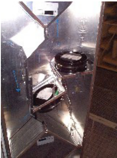
Figure 3 Inside the base station door, showing two fans (from Moorhouse et. al. 2003)
