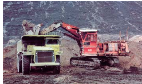
Figure 3. Hydraulic excavator and 77 tonne truck
