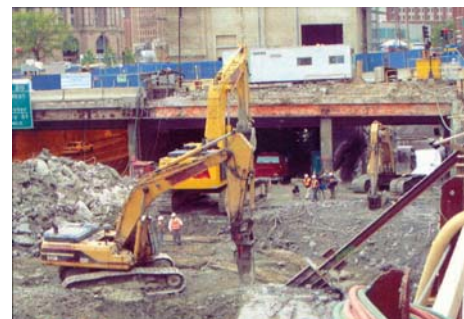
Figure 1. Typical construction equipment
