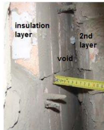
Figure 1: Layered refractory (Palmer, 2008)
