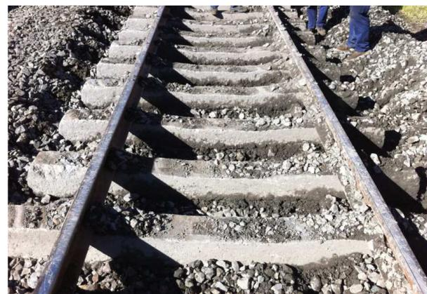
Figure 3. Track damages due to impact loading
