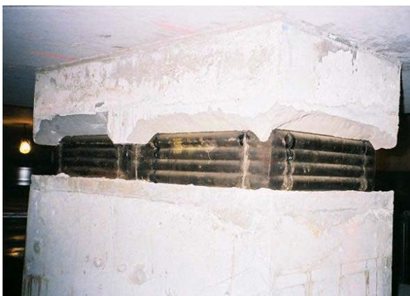
**Figure 9.** Bearing Pads after Installation and Loading
