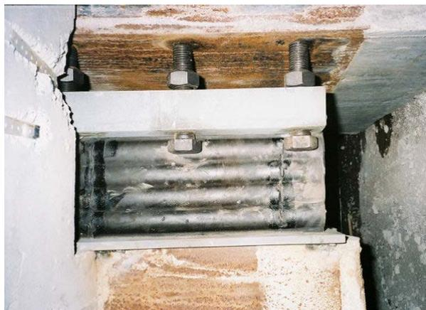
**Figure 11.** Partial View of Lateral Restraint Pad after Compression and Loading
