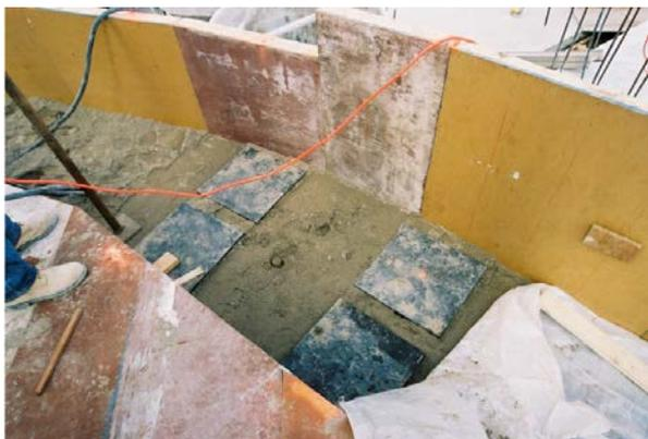
**Figure 8.** Group of Rubber Pads with Sand Filling the Gap between the Support Pads, Prior to Installation of the Top Grout Pads
