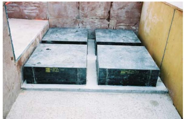
**Figure 7.** Group of Rubber Pads Prior to Pouring Concrete Supporting the Main Hall
