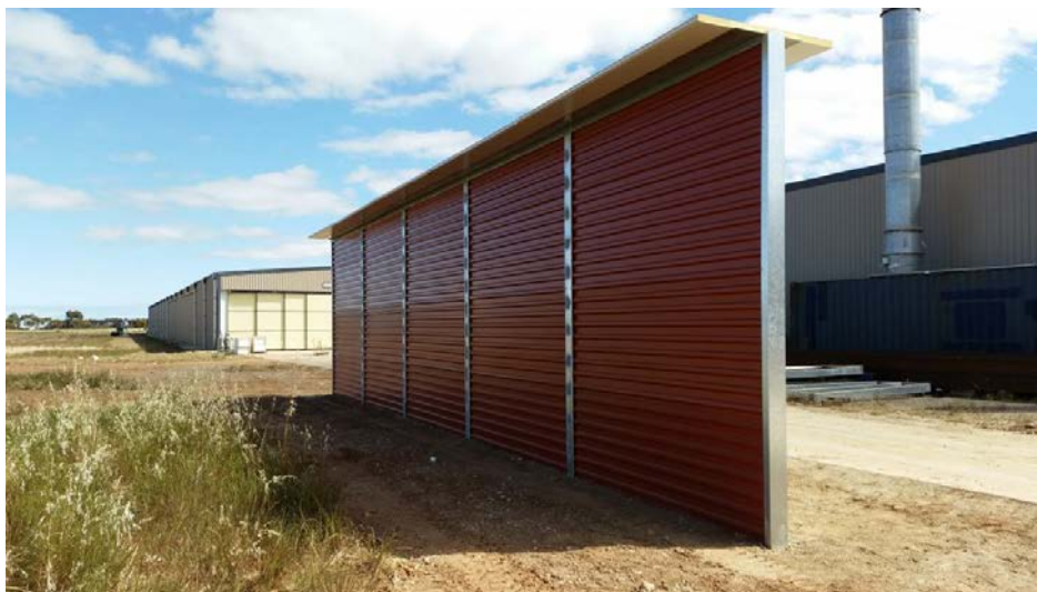
Figure 2. T-profile barrier installed at test site
