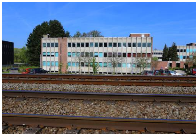
Figure 1: The Block D building is a three-storey building with below-ground basement, located approximately 30 m from the railway track.
