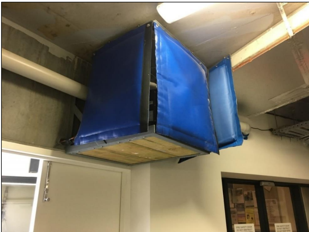
Figure 5 : Figure Illustrating Compressor Enclosure
