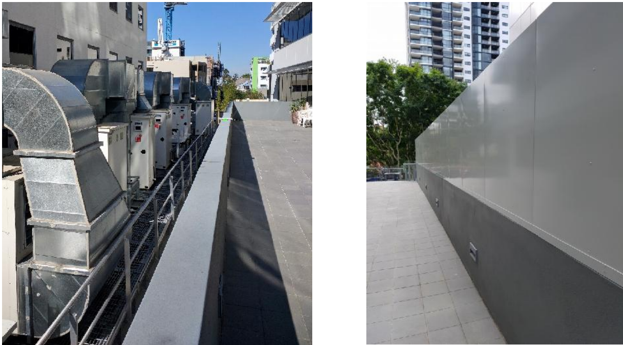
Figure 4: Acoustic Barriers – Before & After
