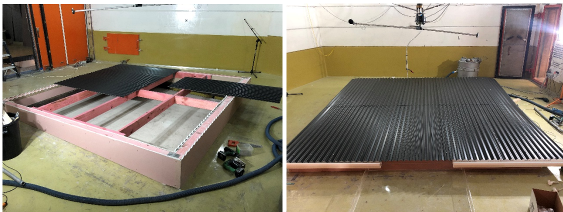
Photograph 3 (left): The test frame during construction, with multiple roofing sheets in place for test fitting Photograph 4 (right): A test system installed, before the addition of polyester insulation into the guttering and reservoir
