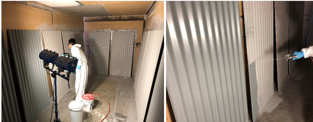
Photographs 1 & 2: Spraying the damping compound onto the corrugated roofing panels
