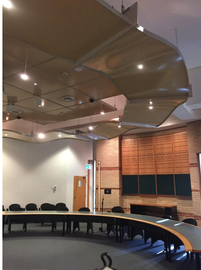
Figure 3: MQU Council Room – existing reflectors and wall panels prior to works
