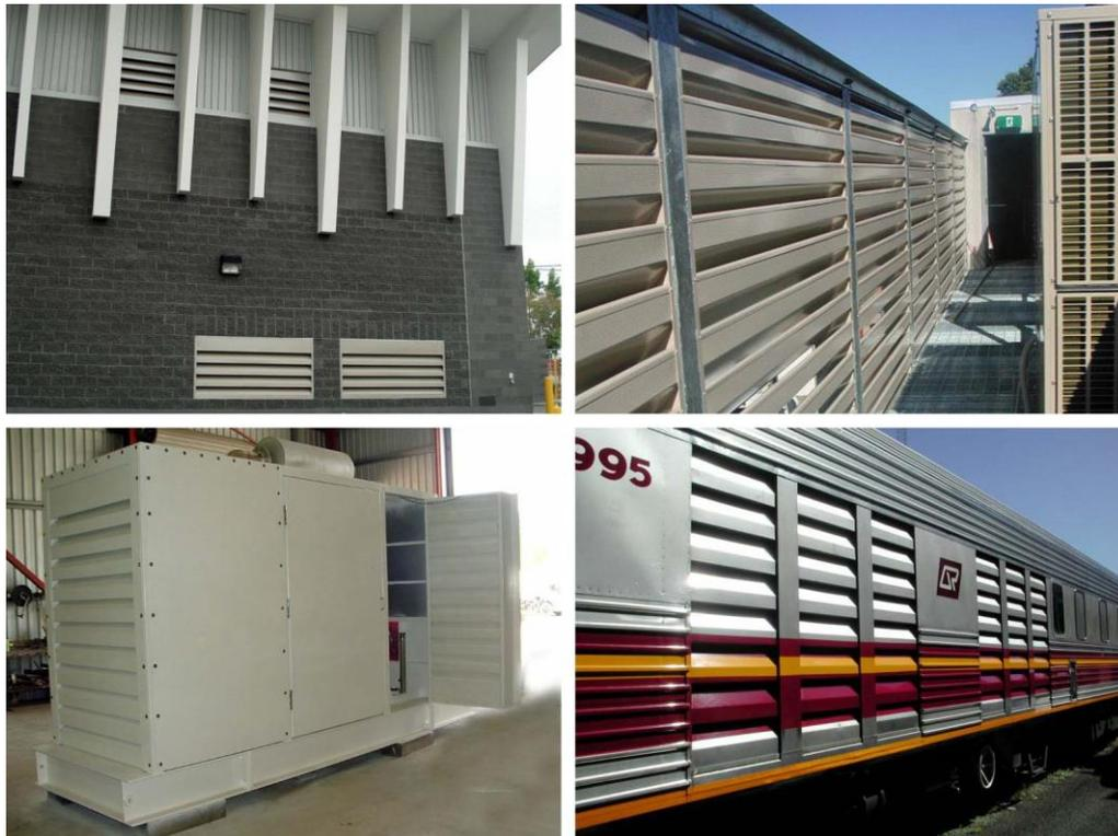
Figure 1: Typical uses of acoustic louvres. Clockwise from top left: Plantroom ventilation, plant deck barriers, mobile equipment and acoustic enclosures.
