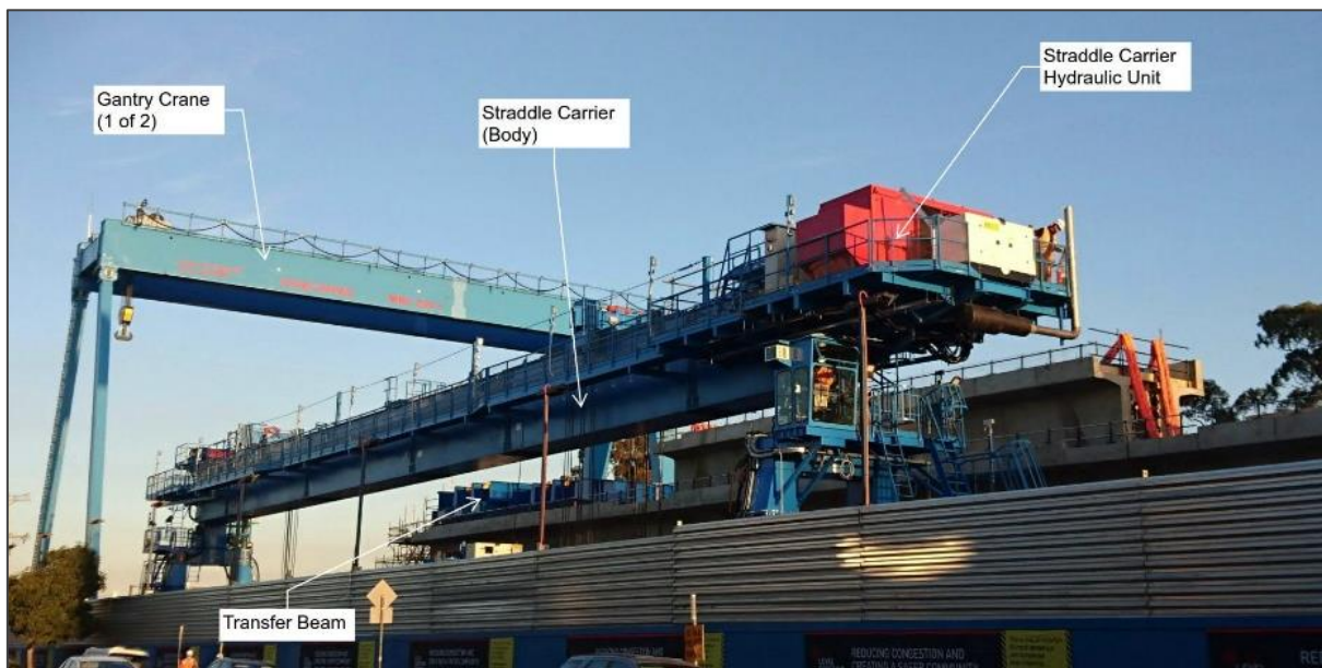
Figure 1: Gantry Crane, Straddle Carrier and Transfer Beam (Support Beam not shown)
