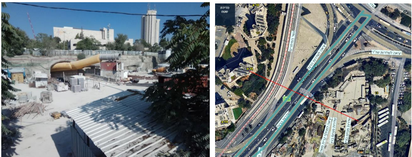
Figure 5: The Fan discharging air from the underground car parking area and the adjacent buildings
