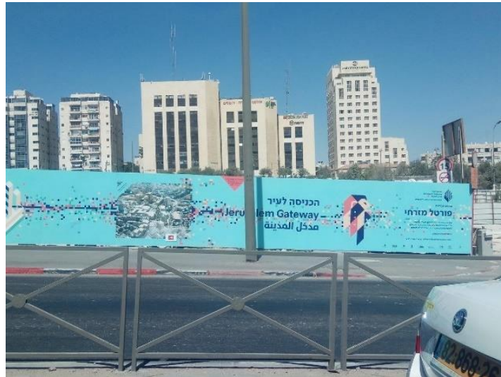
Figure 4: Major Road and Building Construction At the Entrance to the City
