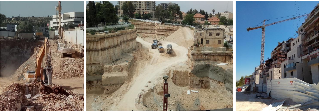
Figure 1: Various construction activities happening around the City
