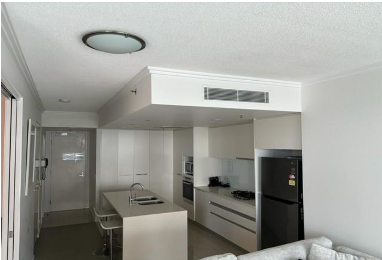
Figure 1 – Stipple finish to the 150mm thick concrete slab ceiling
