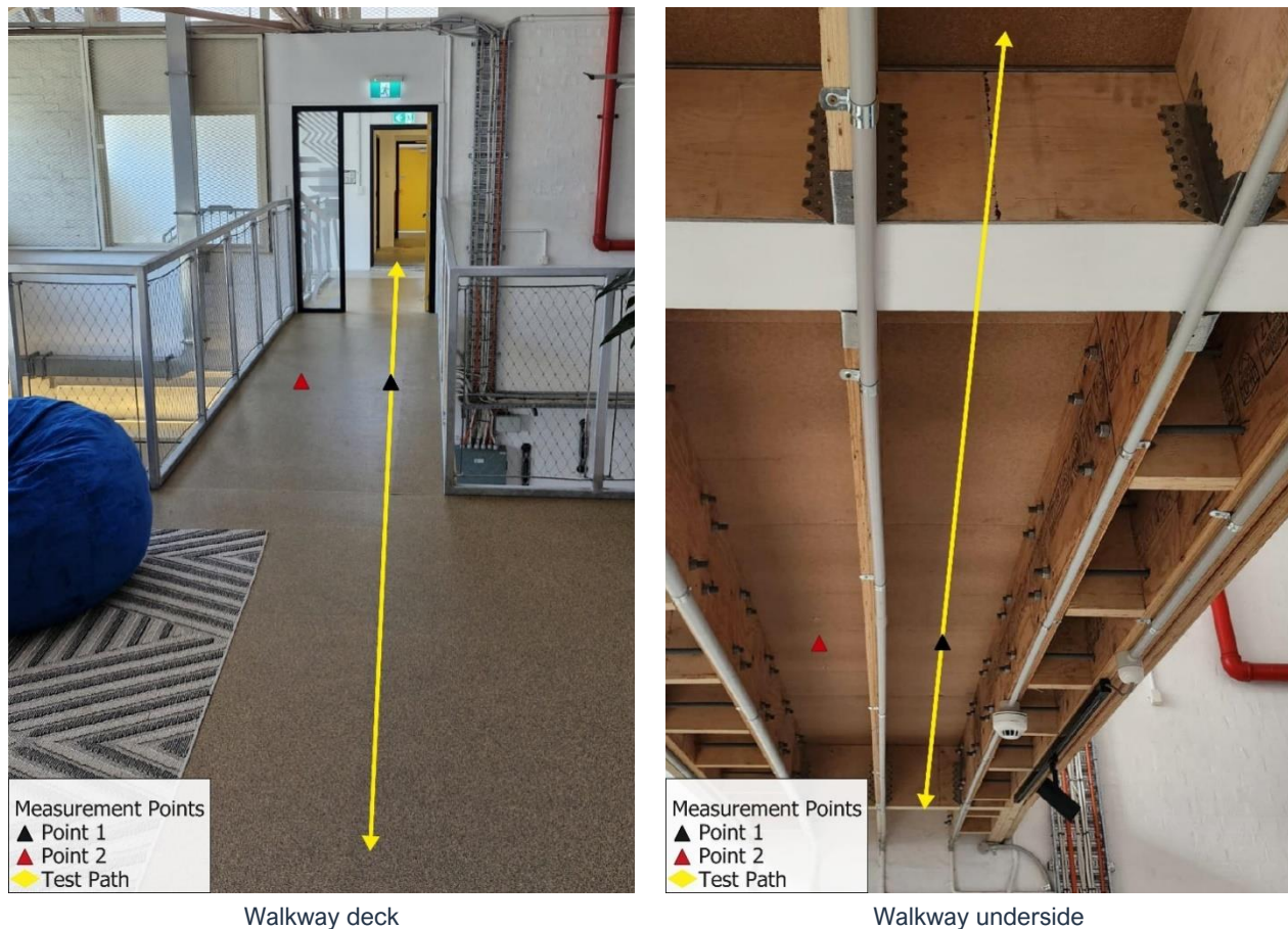
Figure 1 Walking path and walkway.
