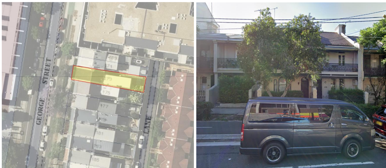
Figure 1 173 George St Redfern is a two-storey terrace house. The airport rail tunnels (dashed line on left image) run underneath George St in front of the property. (image sources: Six Maps and Google Maps)
