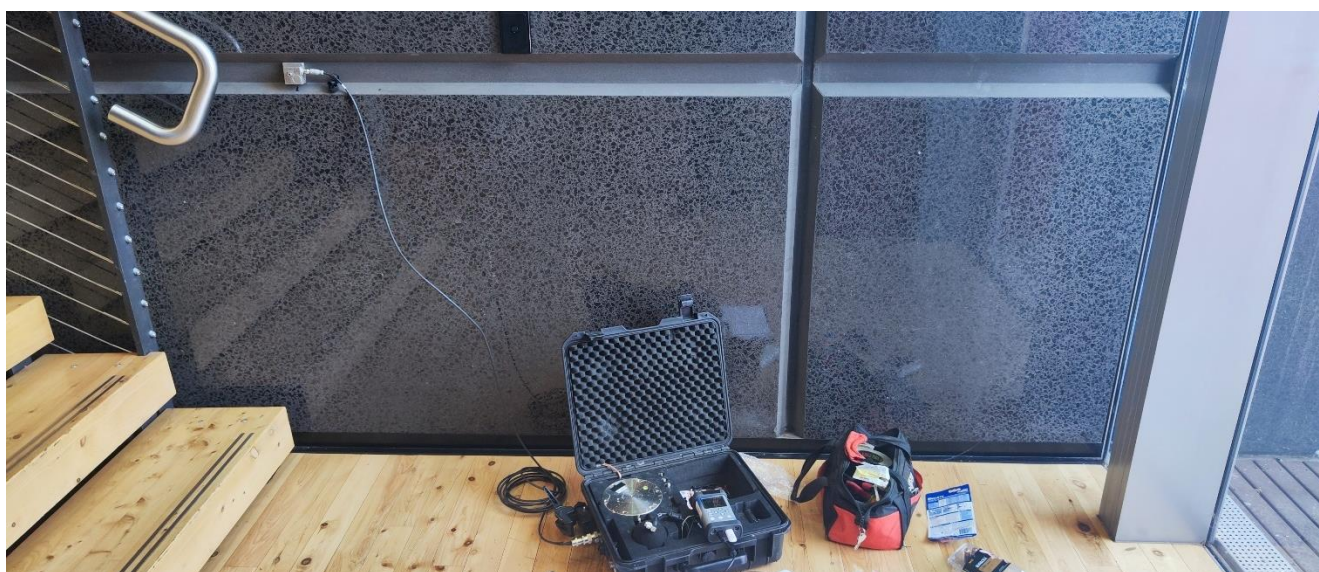
Figure 6 – Accelerometer mounted on the wall in the ground floor lobby, close to the stairwell.
