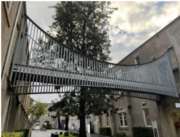
Figure 1 – The Sacred Heart Pedestrian Bridge.
