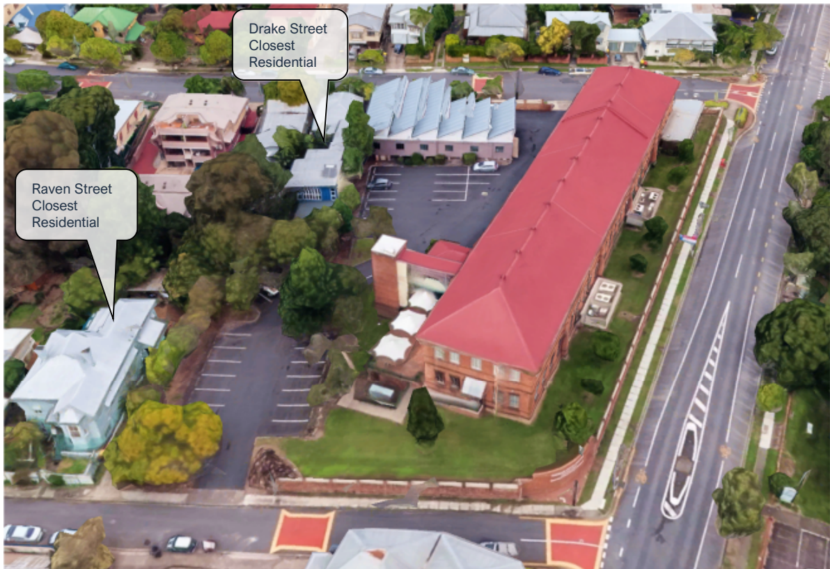
Figure 2 – Overhead View of TDC Pre Refurbishment and Adjacent Residences
