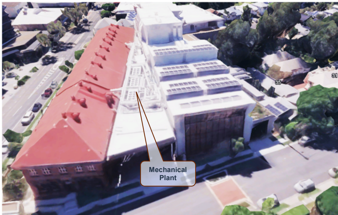
Figure 5 – View showing the Roof Top Mechanical Plant Location
