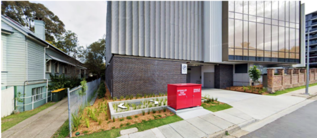
Figure 4 – View showing Closeness of Residence to Rear of Talbot Theatre of TDC Refurbishment
