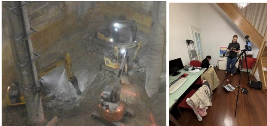
Figures 11 & 12: Construction activities including rockbreaking and excavation (Figure 8) located underneath resident property where attended indirect monitoring took place (Figure 9)
