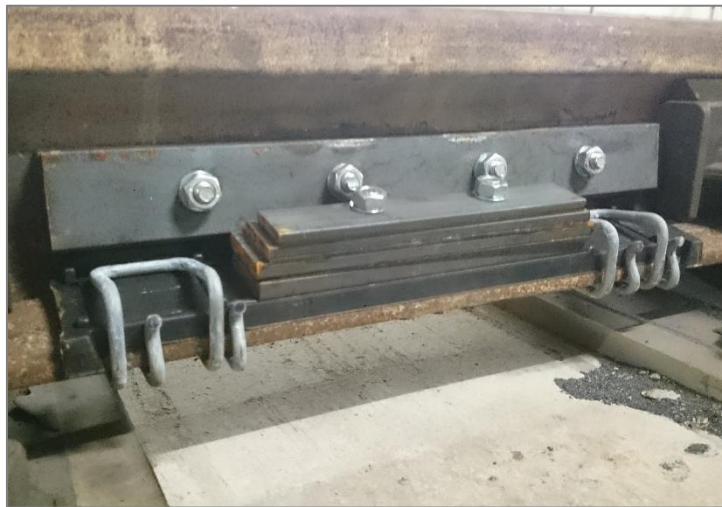
Figure 1: Rail web dampers trialled in Perth Tunnel 6, Fremantle Line up main, 2017.
