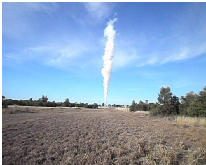
Figure 2 Western Blowdown Vent
