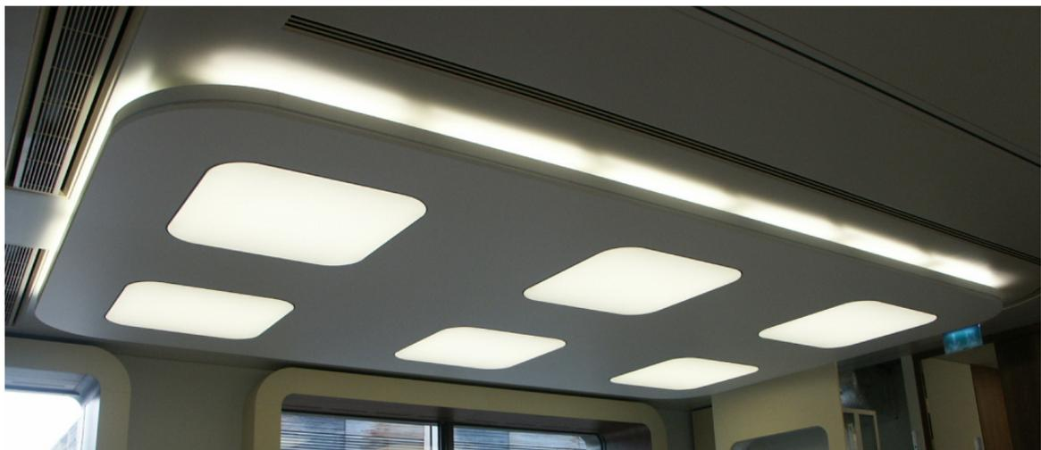
Figure 5: Lighting system/sound absorbing ceiling in an office.
