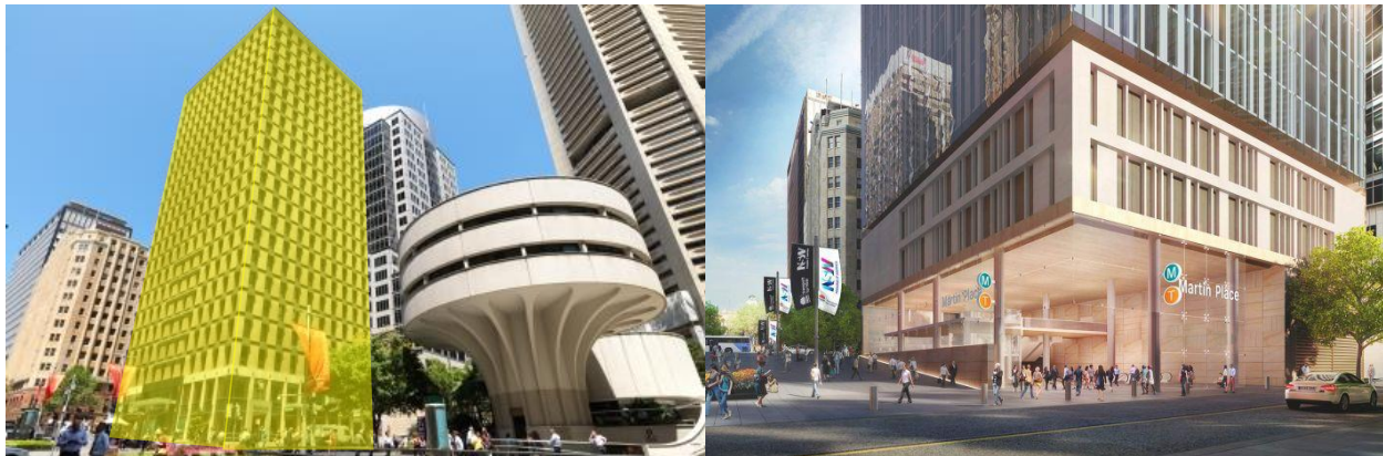
Figure 2: Left: A high-rise building (highlighted) to be demolished to make way for the new Martin Place metro station in Sydney. Right: An artist's impression of the new station (with over-station development above)
