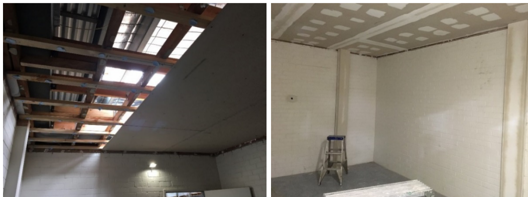
Photograph 1 and 2: Construction of the reverberation room ceiling
