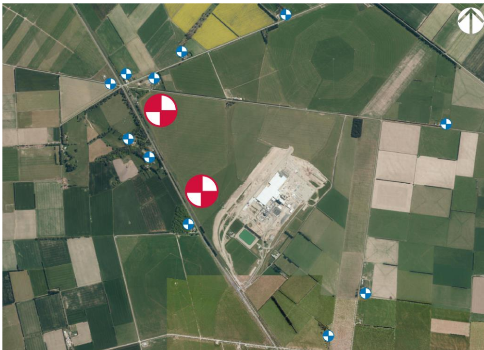
Figure 4 –Darfield site with Stage 2 under construction and alternative locations marked in red and dwellings in blue.
