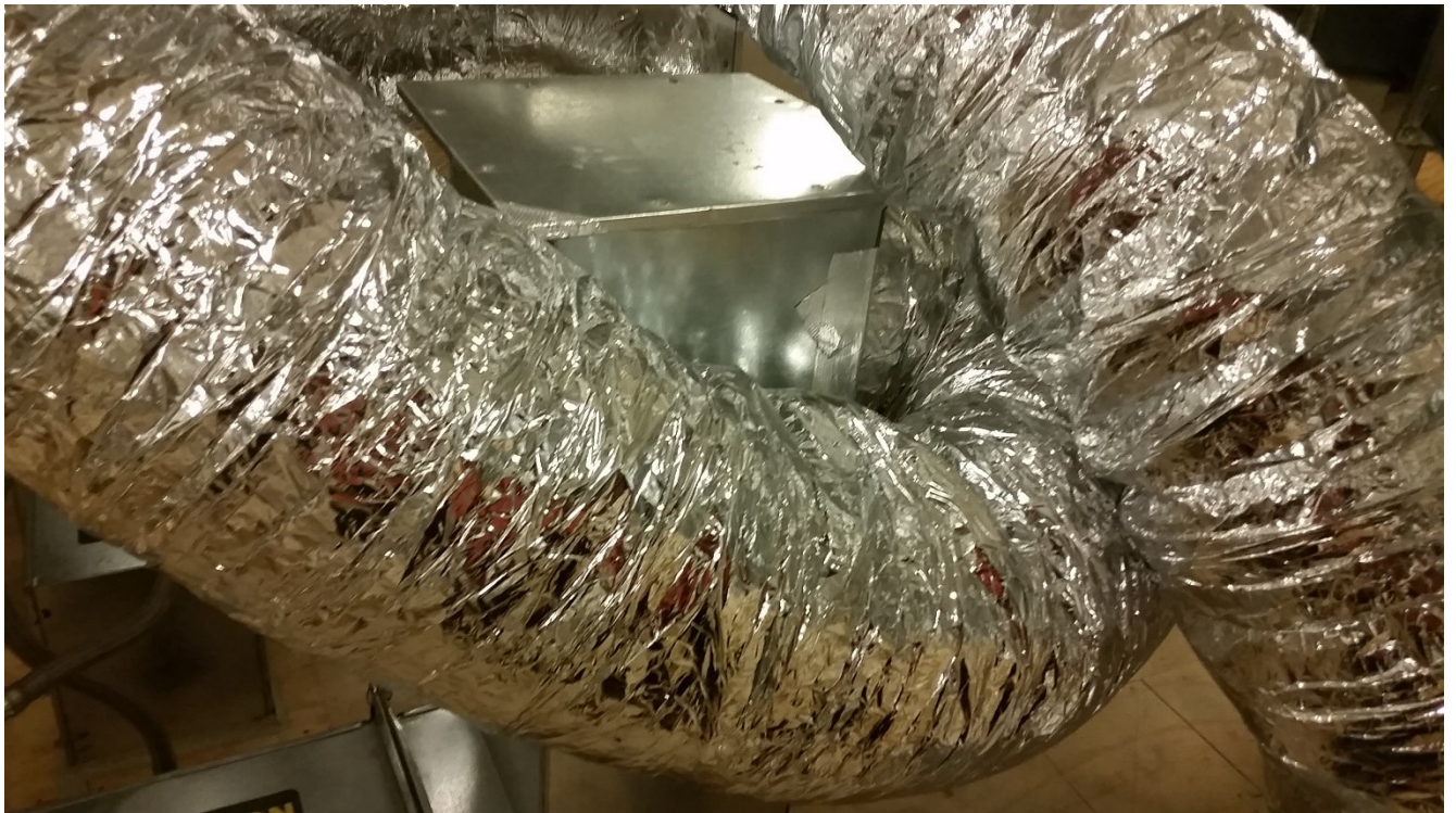
Figure 3: Poorly-aligned flexible ductwork caused high aerodynamic noise levels and required modification
