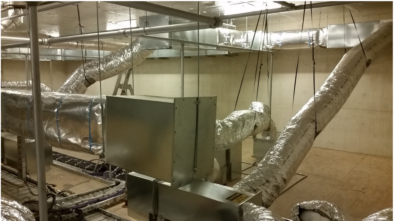
Figure 4 Flexible ductwork required additional support from straps to keep the required duct routing
