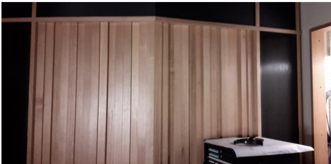
Figure 6 Angled rear wall used to achieve 15 ms ITDG in small control rooms
