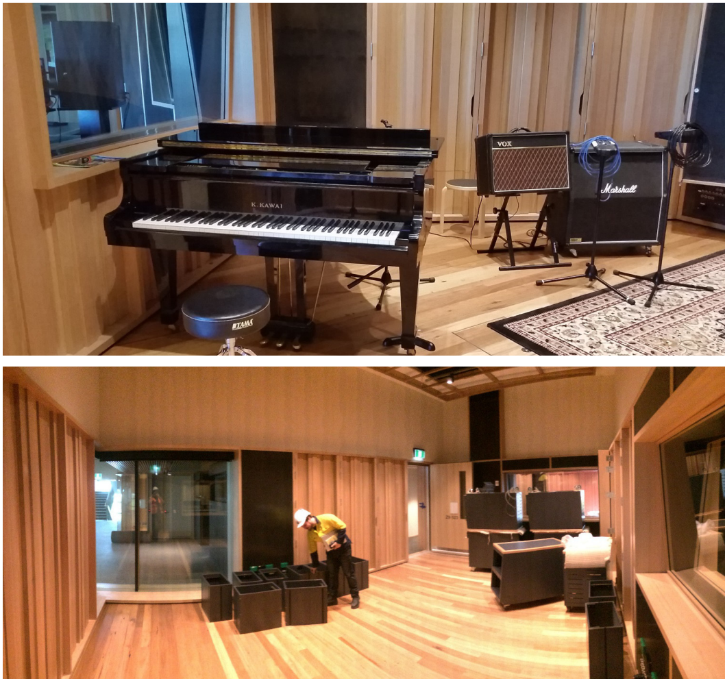
Figure 10 Views of Recording Studio Live Rooms, showing hinged reversible panels and room finishes
