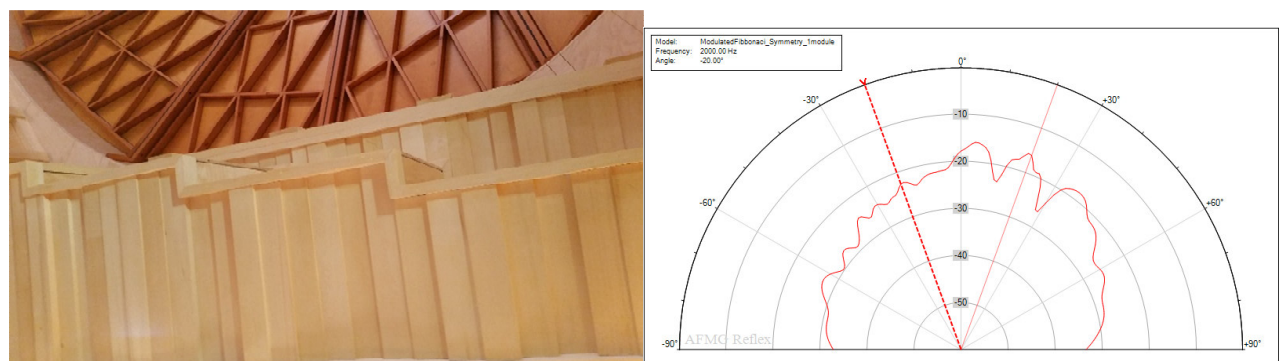
Figure 10 Soffit Diffusion image and Spatial Response (2 kHz)
