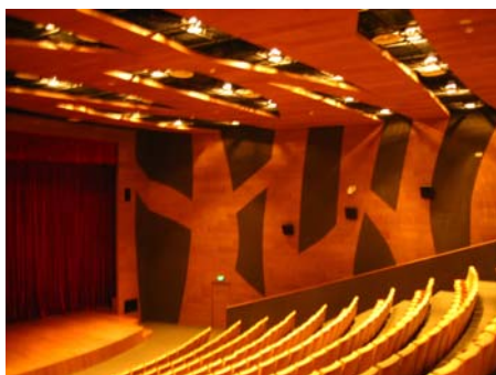
Fig.10 Photograph of cinema auditorium utilizing W-MPP
