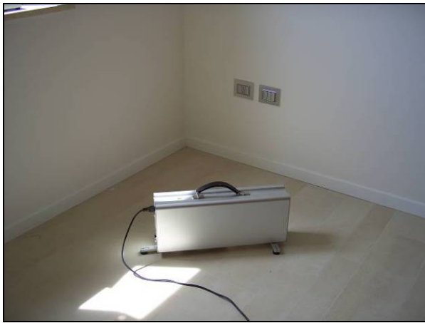
Figure 4. Case study: in situ measurement of weighted normalized impact sound pressure level of floors L'_{n,w}
