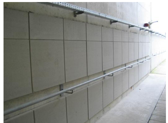
Reapor Installed in tunnel
