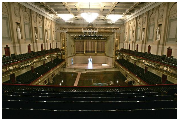
Figure 2: Boston Symphony Hall. The stage house is high, wide, and shallow, with sloping side walls and ceiling. Reflections from these surfaces are directed into the hall, and multiple reflections do not occur within the stage house. Instruments in the rear of the orchestra have equal clarity as instruments in front. Notice the coffers on the ceiling, and the niches along the side walls.
