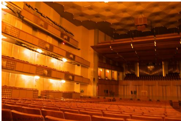
Figure 4: The Kennedy Centre, Washington, DC. Note the flat canopy over the orchestra, and the rippled – not coffered – ceiling in the hall. No niches or coffers adorn the side walls. The audience on the stage absorbs some of the sound that would otherwise go to the hall. The sound in the first half of the stalls is not as loud as Boston, but reasonably clear. The author has not heard the sound further back.
