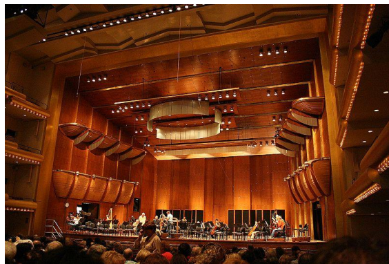
Figure 1: Avery Fisher Hall, New York City. Note the deep, low ceilinged stage house, with nearly parallel side walls. These surfaces trap sound inside the stage, which scrambles the phase coherence of the harmonics from instruments in the rear of the orchestra. The ceiling of the hall is basically flat, as are the side walls.
