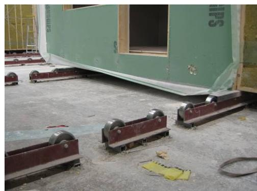
**Figure 4.** The volumes are supported with moving rails on the floor
