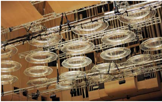
Figure 14. Existing cloud canopy, temporarily reconfigured on tri-truss
