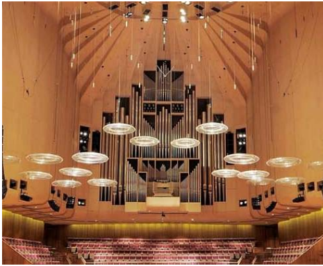
Figure 5. Existing acoustic reflectors, known as 'clouds'
