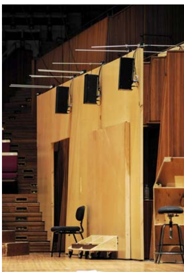
Figure 16. Prototype flat MDF wall panels
