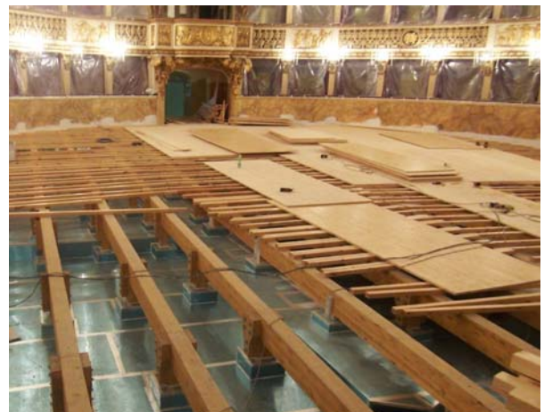
Figure 3. Wooden floor construction in the stalls area
